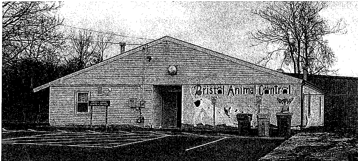
Figure 1-Front view of existing building
