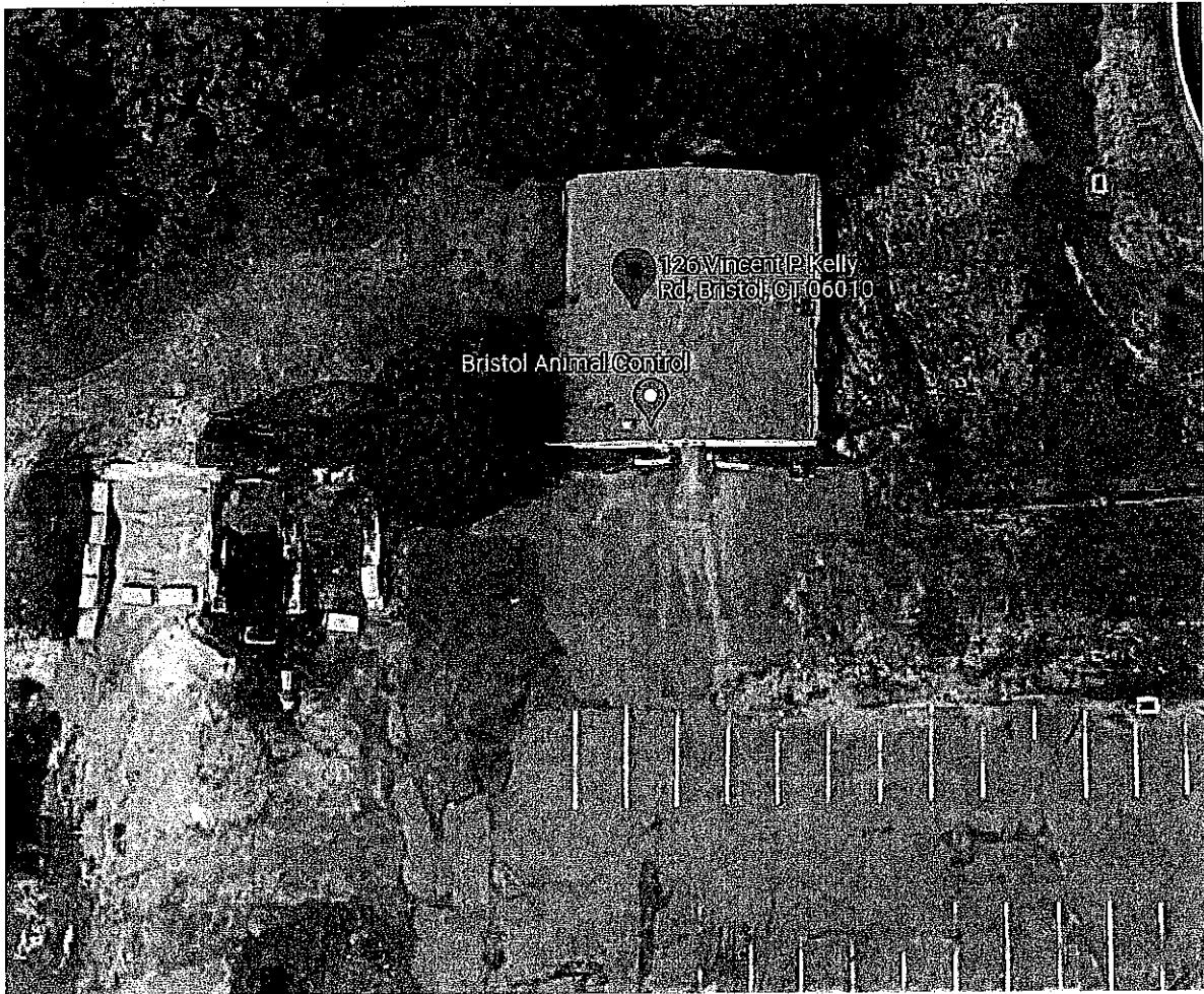
Photo 1-Aerial View of existing building
