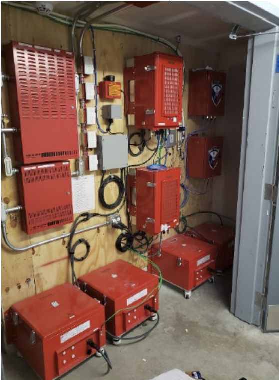
VHF/UHF System (requires more space in head-end room)
