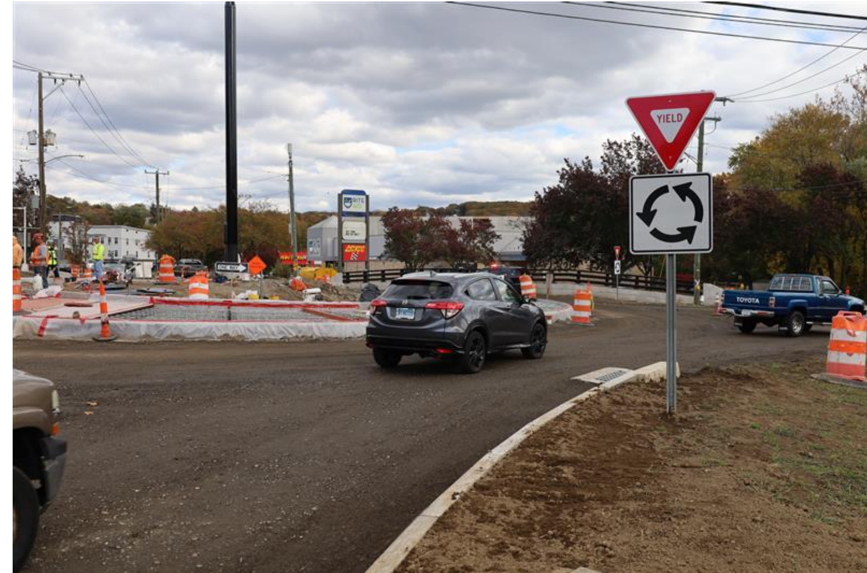
LOTICIP funded roundabout – Naugatuck, CT
