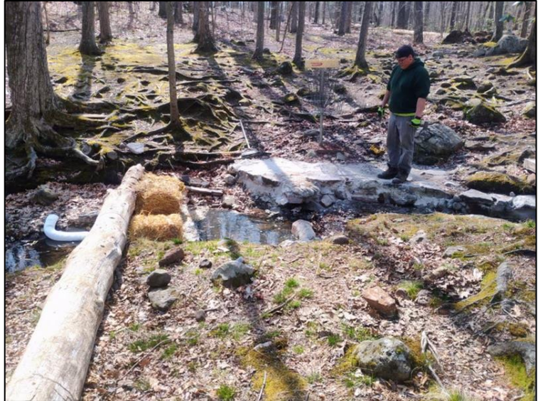
Figure 2. Installation of watercourse protection measures.
