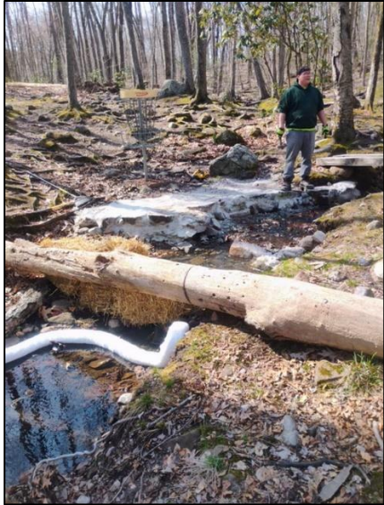
Figure 1. Installation of watercourse protection measures.
