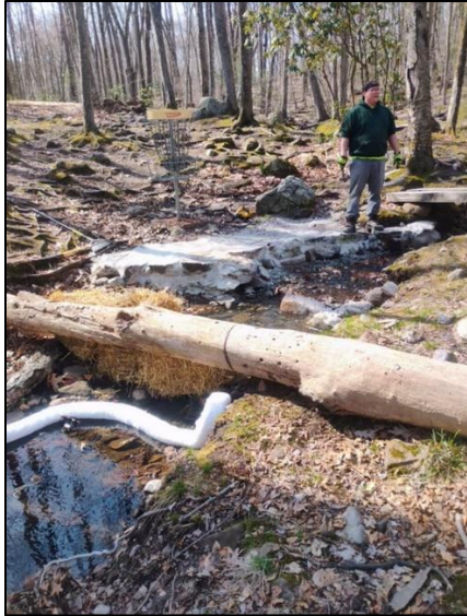
Figure 1. Installation of watercourse protection measures.
