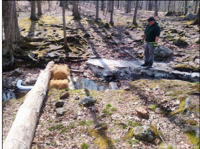
Figure 2. Installation of watercourse protection measures.
