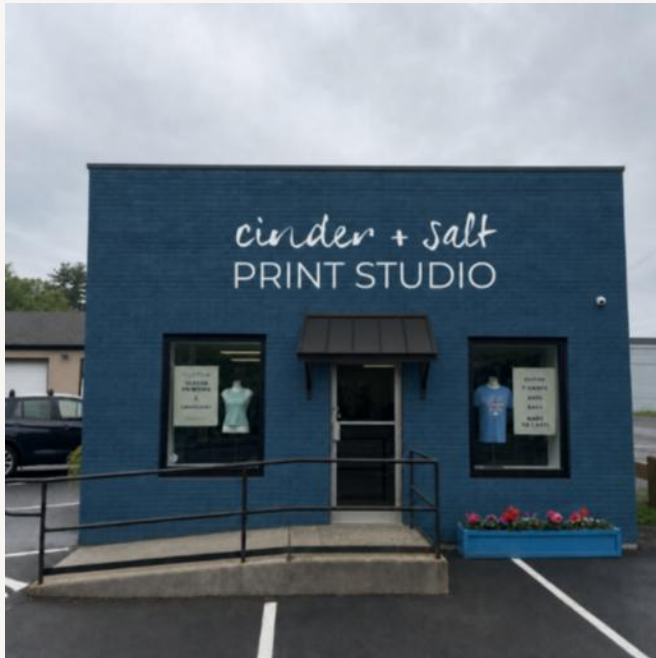
Front of Building
