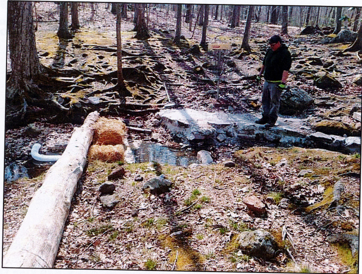
Figure 2. Installation of watercourse protection measures.
