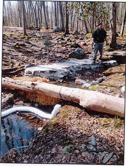
Figure 1. Installation of watercourse protection measures.
