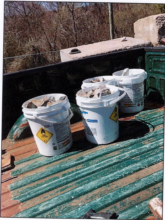
Figure 3. Removed cement from the streambank.
