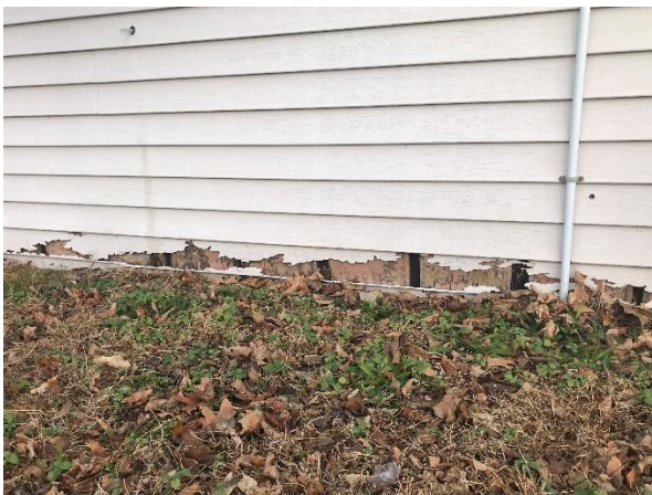
Photo 2-Siding Damage
