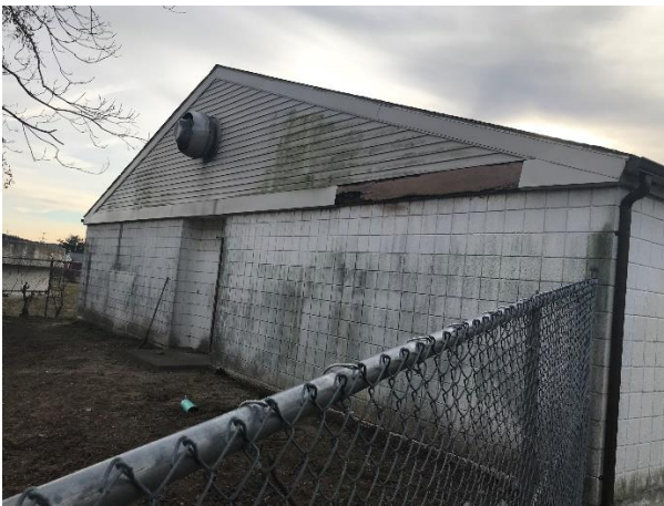
Photo 6-Siding Damage
