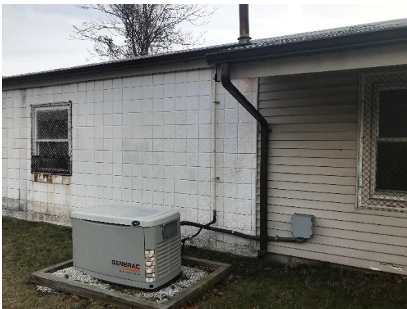
Photo 12-Gas Fired Generator
