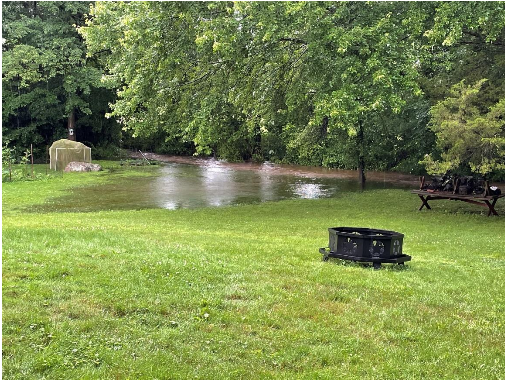
Figure 35: Stormwater Overtopping Channel Banks
