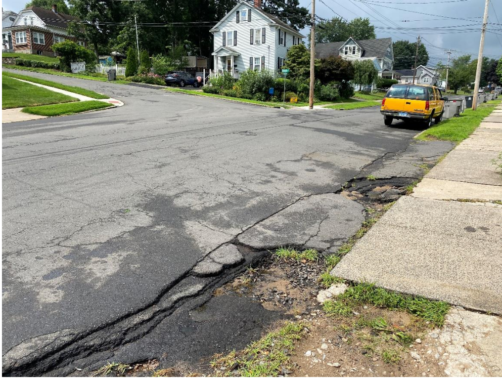
Figure 12: Driveway Apron Looking Toward Melville Street
