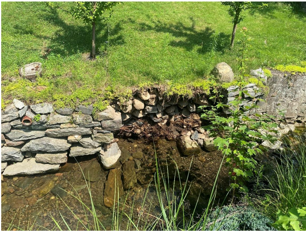
Figure 18: Channel Wall Adjacent to 90 Field Street
