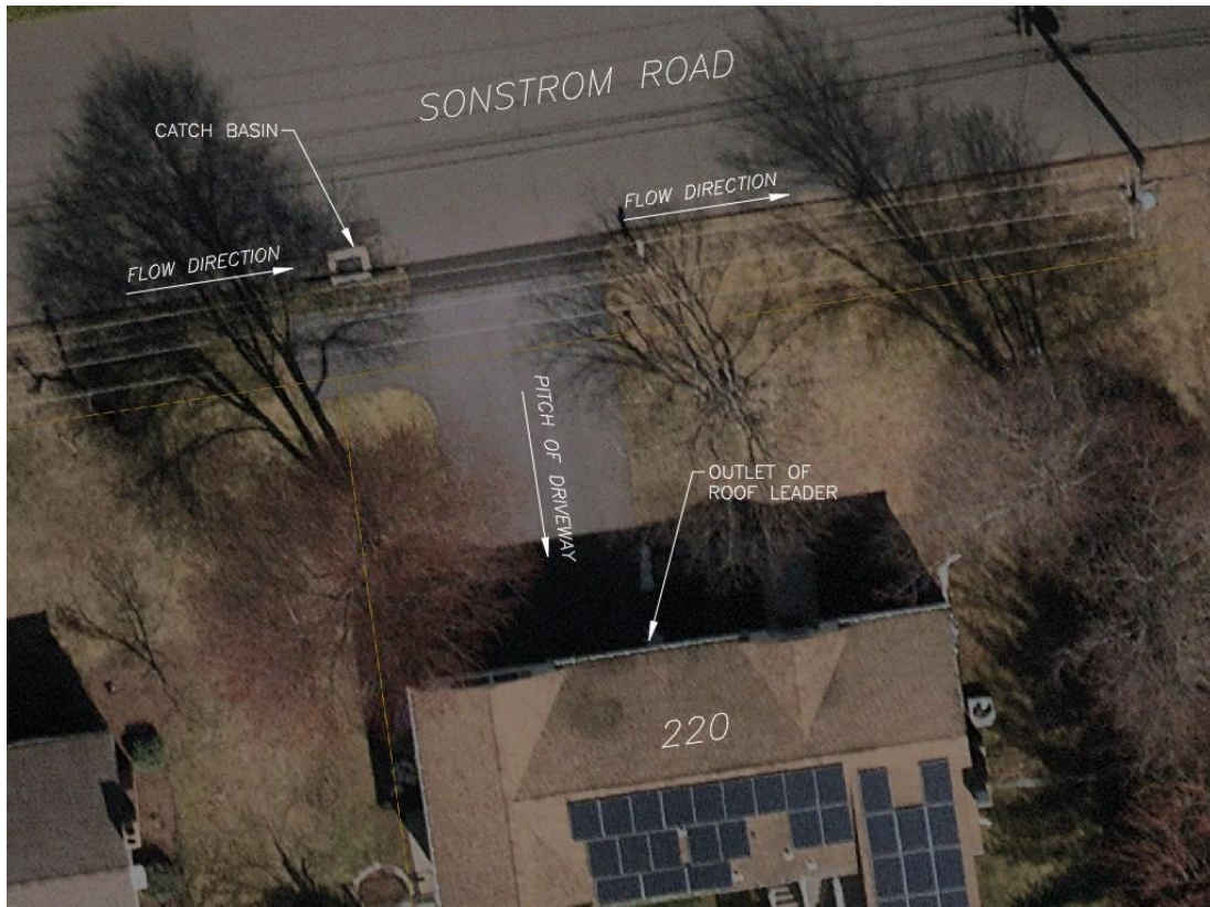
Figure 23: Site Conditions at 220 Sonstrom Road
