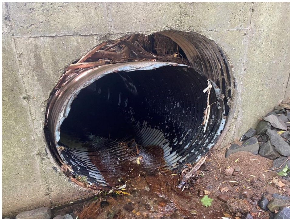
Figure 10: Downstream Culvert on Private Property
