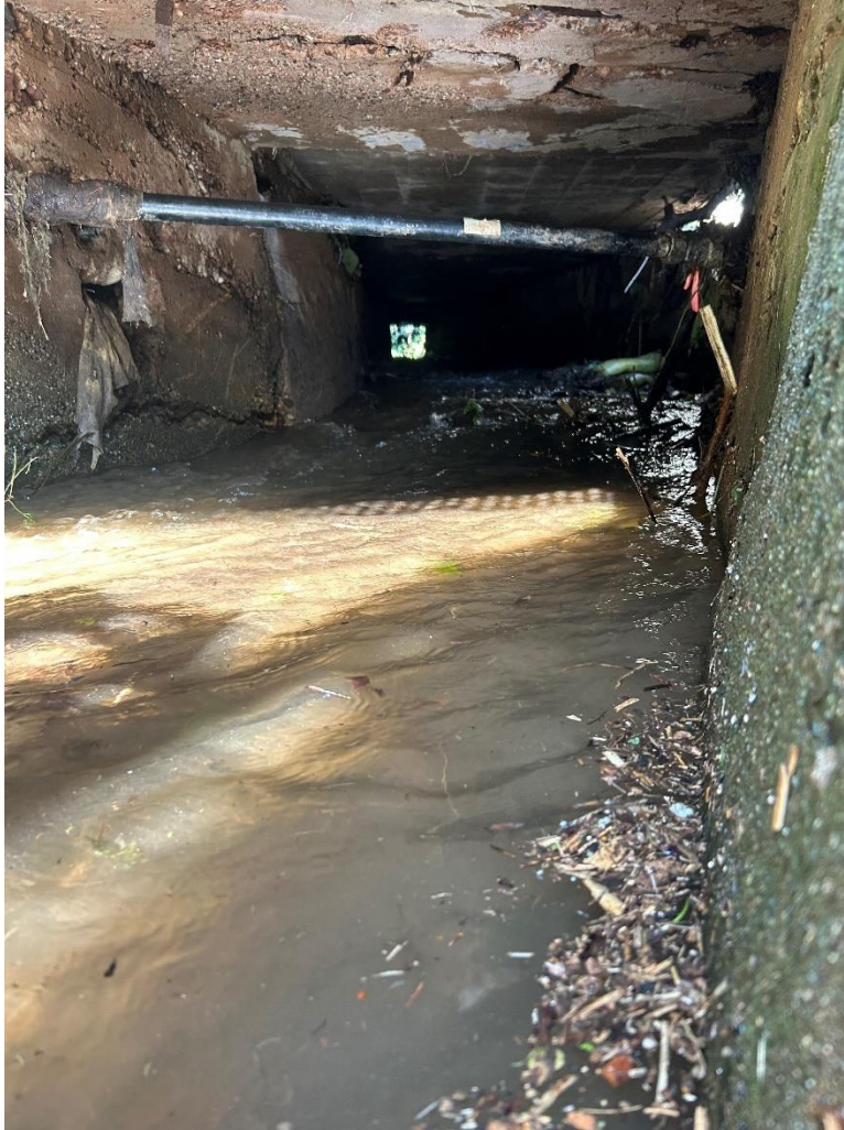
Figure 69: Private Culvert Cleared of Debris
