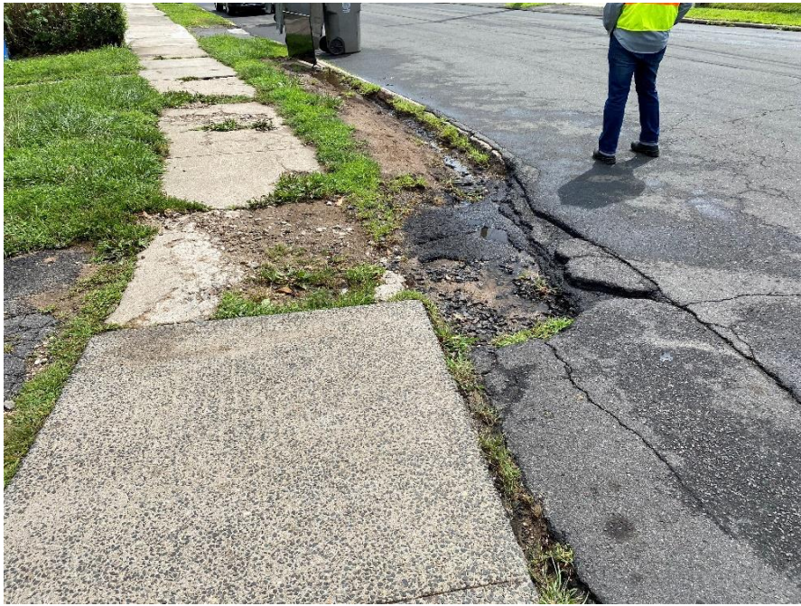
Figure 19: Existing Conditions Before Reconstruction
