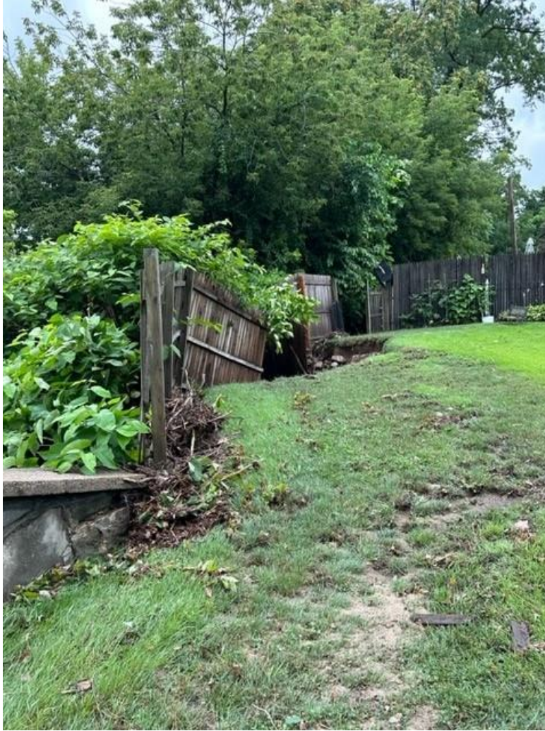
Figure 64: 316 Divinity Street Property Damage
