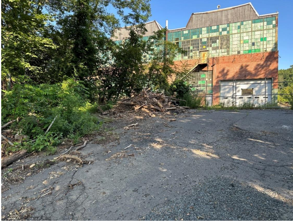
Figure 60: Debris Removed from Channel
