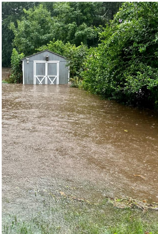
Figure 13: Floodwaters at 114 Blakeslee Street
