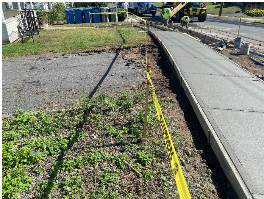
Figure 20: Reconstruction of Sidewalk and Curbing
