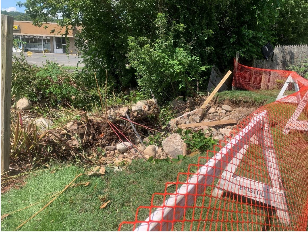
Figure 65: 316 Divinity Street Property Damage
