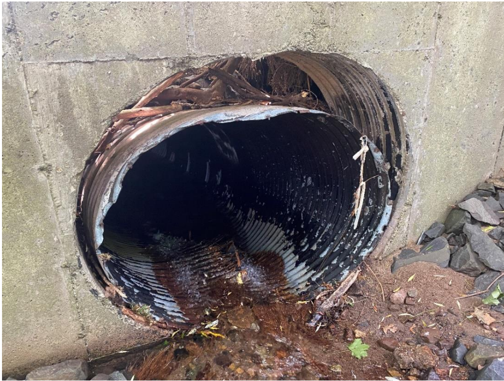
Figure 14: Downstream Culvert on Private Property
