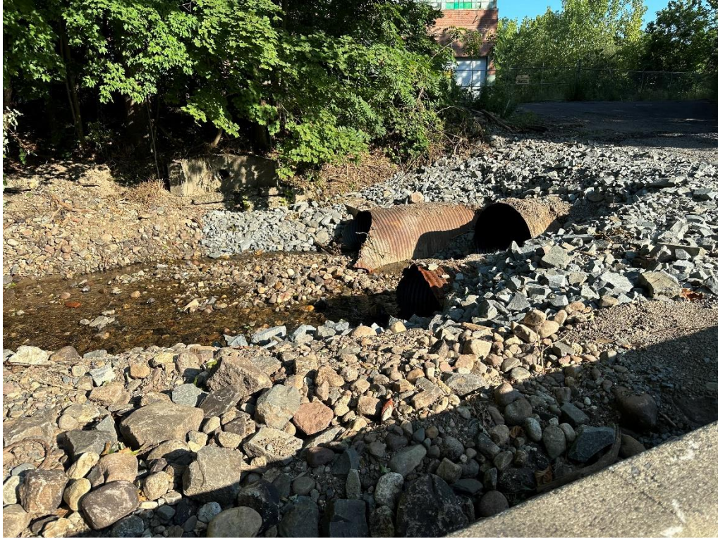
Figure 58: James Street Culvert
