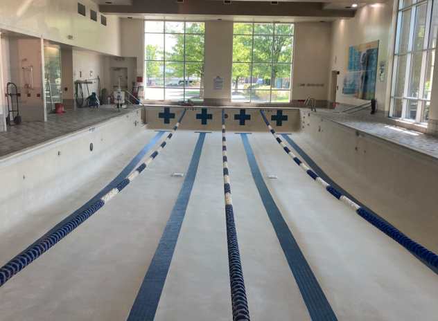
The empty pool at the former LA Fitness will reopen as a saltwater pool when GA Fitness takes over the building.
