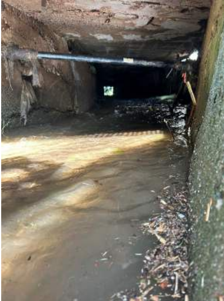
Figure 68: Private Culvert Cleared of Debris
