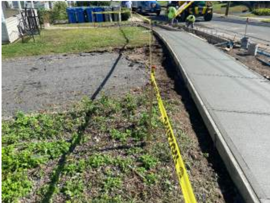
Figure 19: Reconstruction of Sidewalk and Curbing
