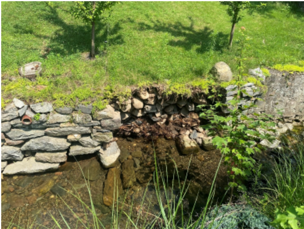
Figure 24: Channel Wall Adjacent to 90 Field Street
