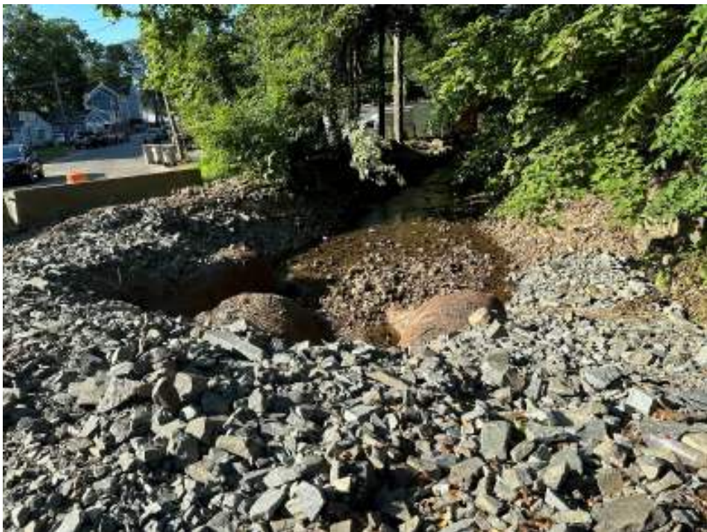
Figure 58: Channel Looking Downstream
