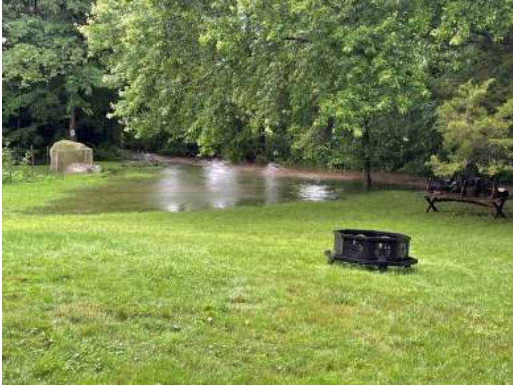
Figure 43: Stormwater Overtopping Channel Banks
