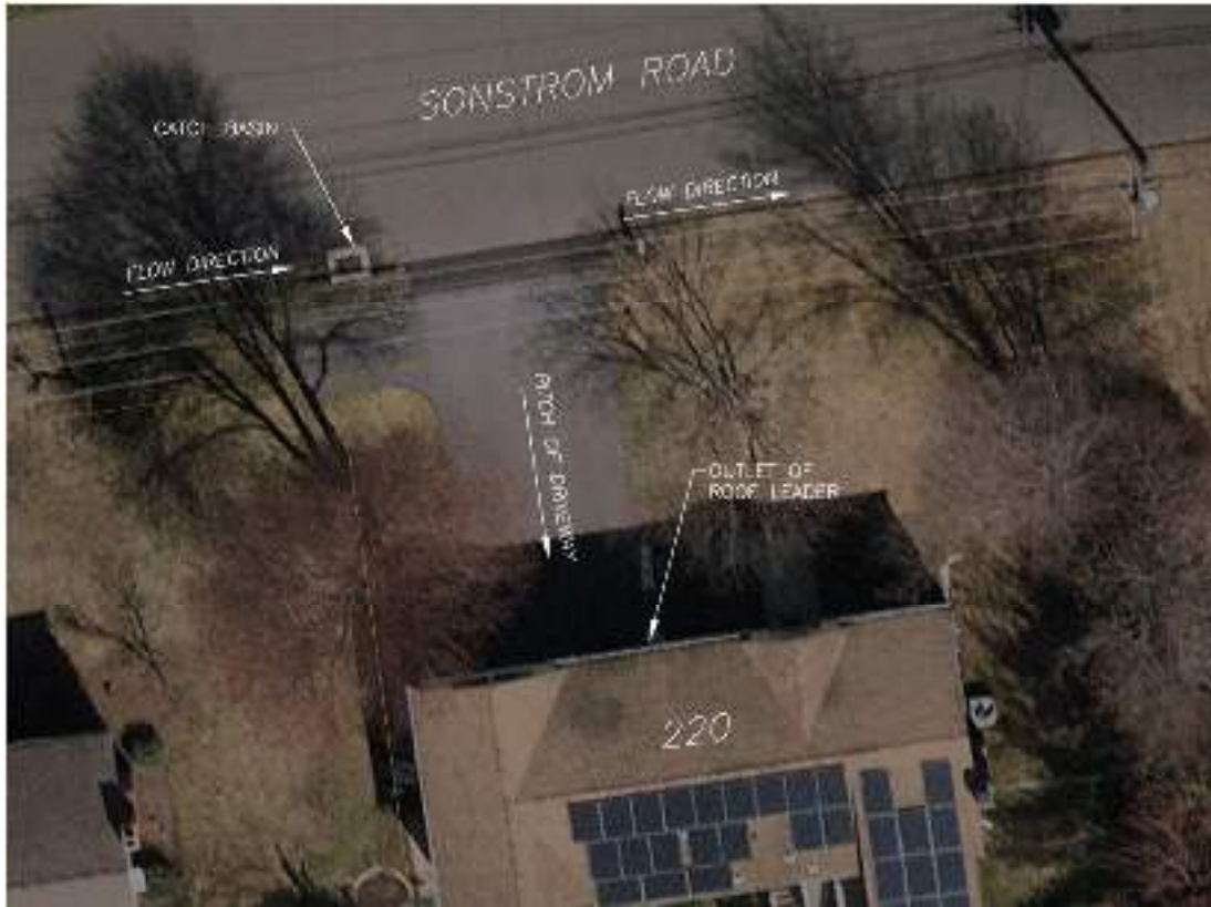
Figure 29: Site Conditions at 220 Sonstrom Road
