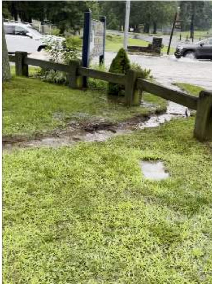
Figure 73: Swale Cut Along King Street
