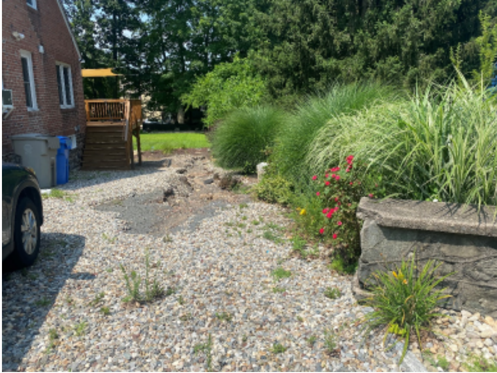
Figure 23: Erosion of Unpaved Driveway
