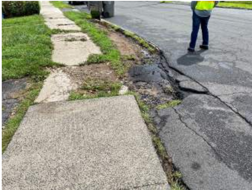
Figure 18: Existing Conditions Before Reconstruction
