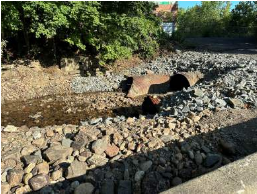
Figure 57: James Street Culvert
