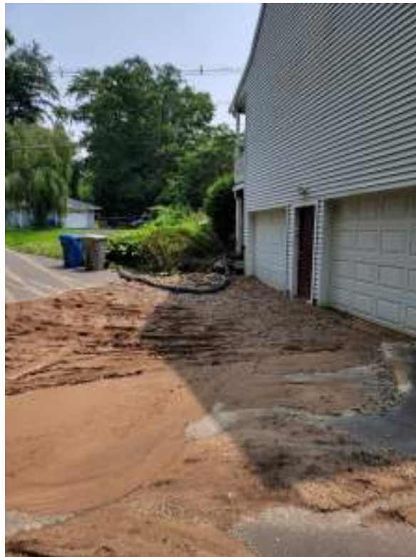
Figure 49: Deposits of Eroded Material
