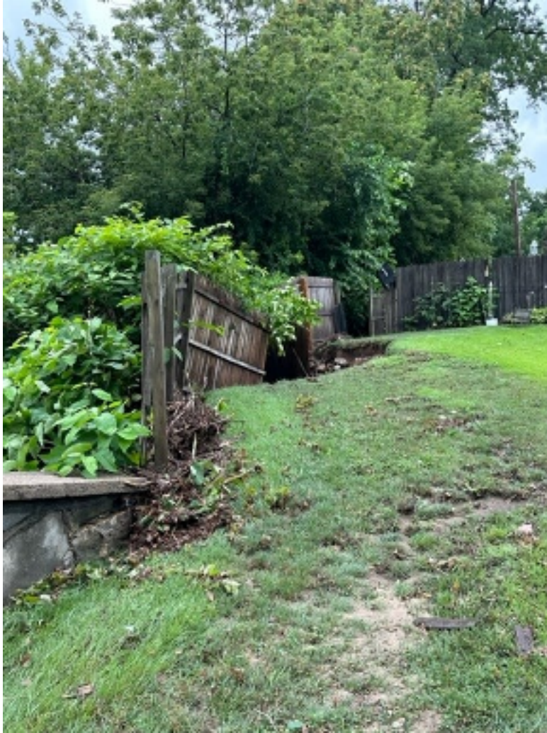
Figure 63: 316 Divinity Street Property Damage
