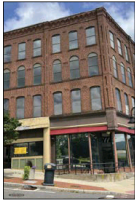
Dylan Braccia The historic building at 238 Main and 13 Prospect streets was approved to allow for a self-storage facility in downtown Bristol.
