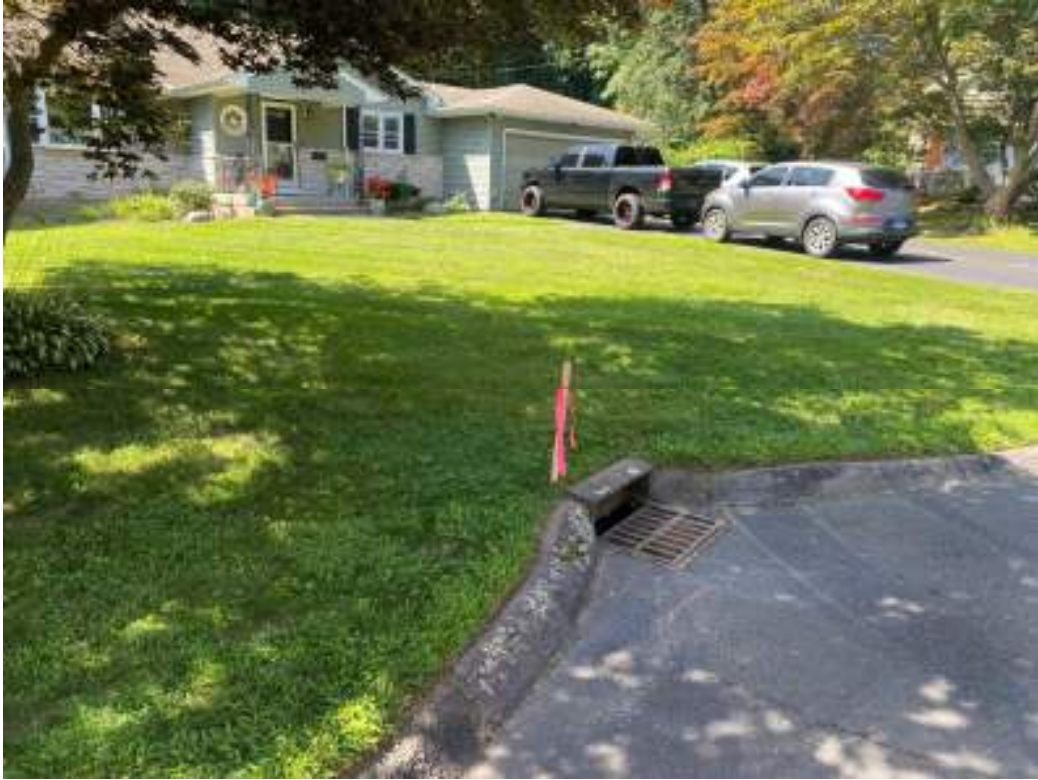
Figure 10: Substandard Catch Basin To be Replaced
