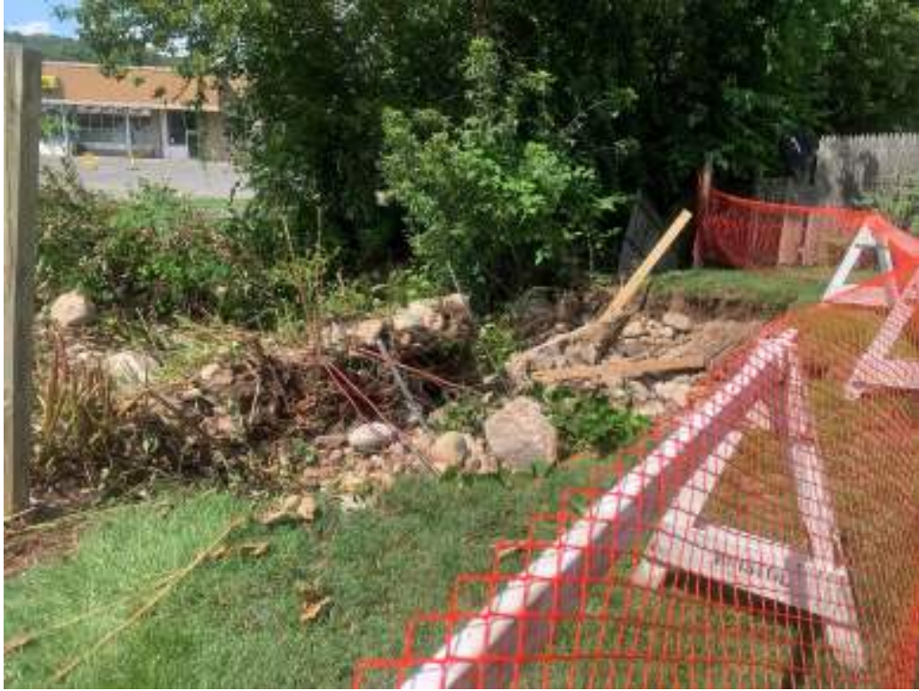
Figure 64: 316 Divinity Street Property Damage
