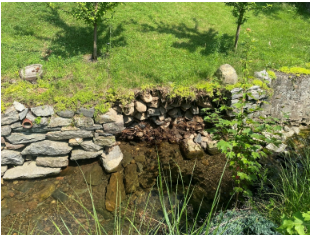
Figure 24: Channel Wall Adjacent to 90 Field Street
