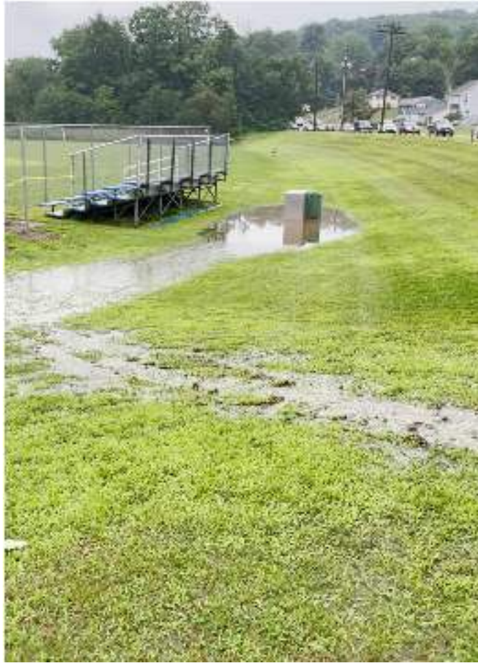
Figure 72: Ponding at Page Park
