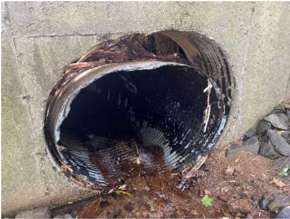
Figure 13: Downstream Culvert on Private Property
