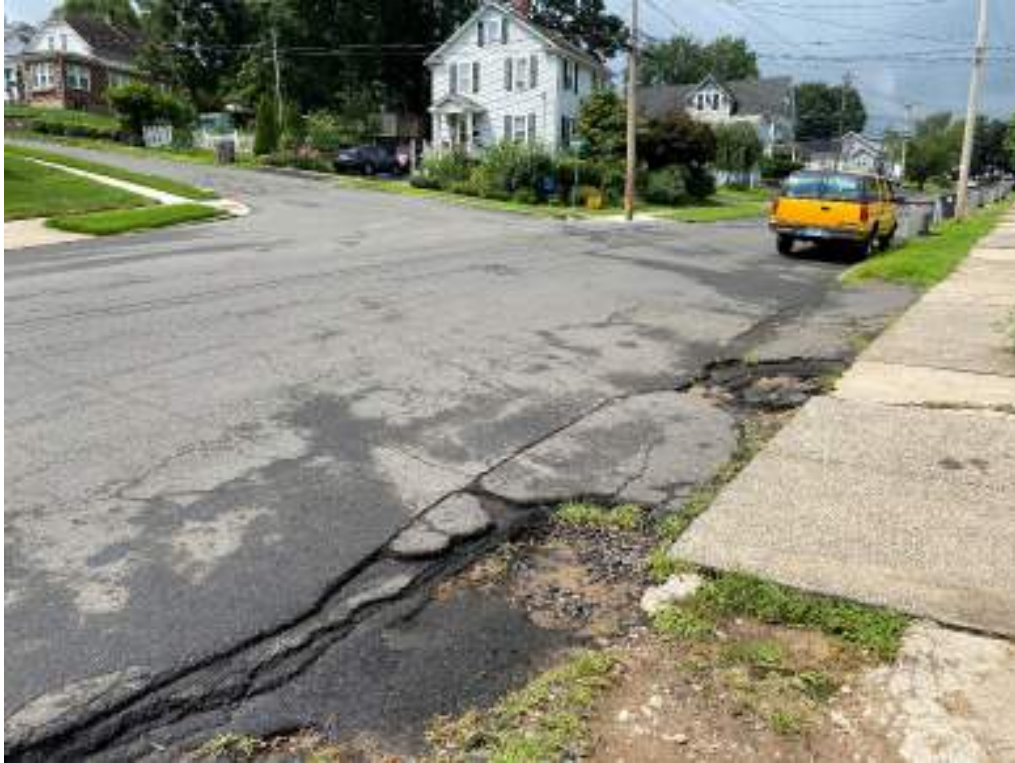
Figure 16: Driveway Apron Looking Toward Melville Street
