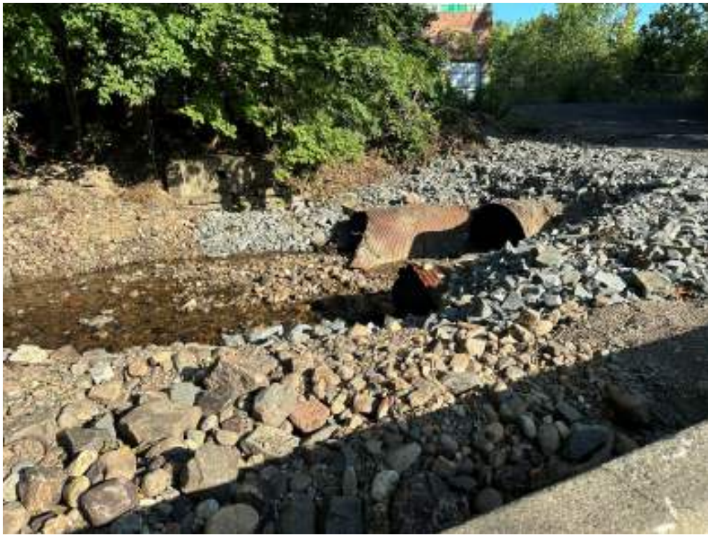
Figure 57: James Street Culvert
