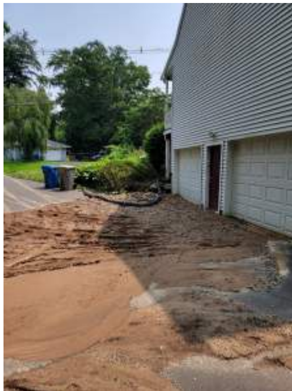
Figure 49: Deposits of Eroded Material
