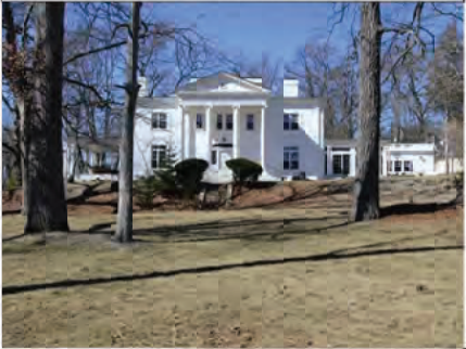
161 Grove St - Chimney Crest (1918) 4,762 SF Colonial Revival, Portico, Veranda, sym. entry, Stone wall / shared boundary, Architect: Walter P. Crabtree
