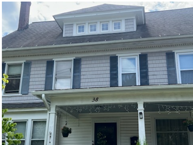
Photo of front of house before replacement
