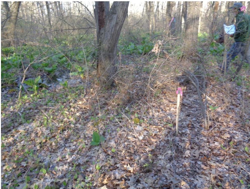
Stake, identified as overflow weir, looking toward south property
