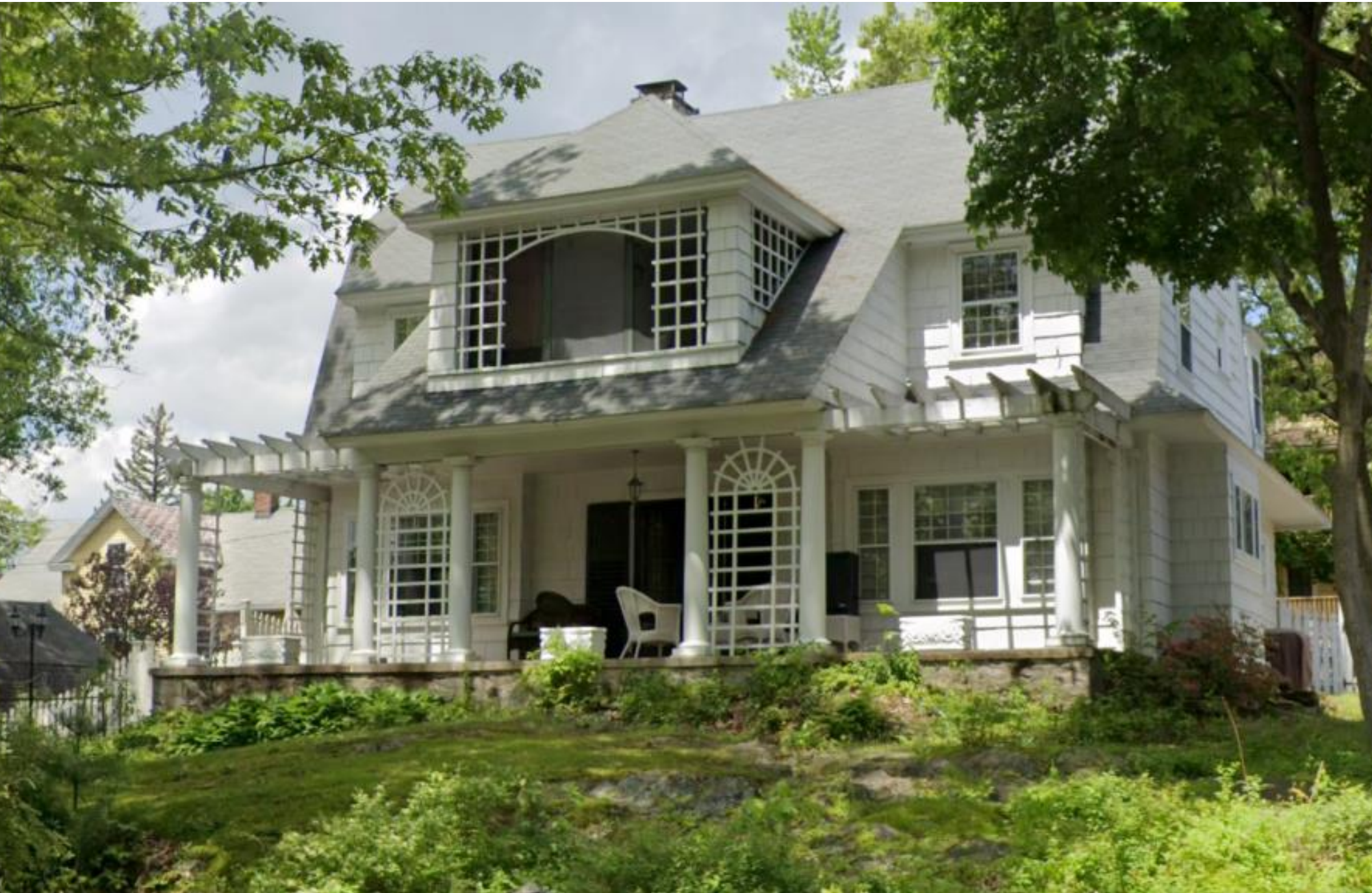
Google Street View – 17 Broadview Street (2019)
