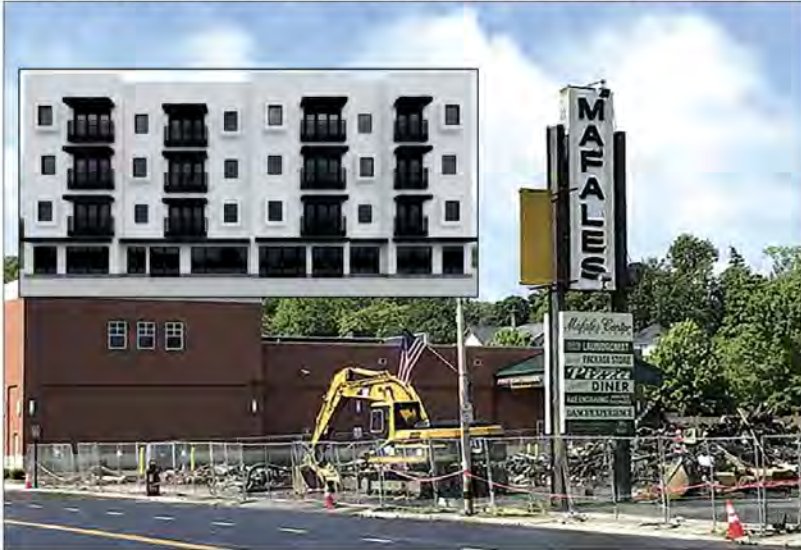
A file photo shows the remains of the Mafale's Plaza at 37 Main St. after a fire in 2022. (Inset) A rendering by architect Schadier Seinau Associates P.C. showing the four story, mixed-use building planned for 37 Main St.
