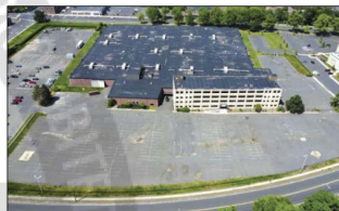
The former Associated Spring complex located at the corner of Main Street and Memorial Boulevard in Bristol.
