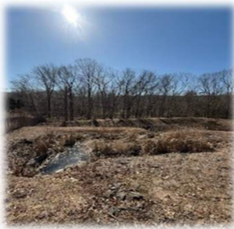
Photo: Tyler Way pond, forebay vegetation
