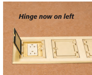
Rotate and reinstall cover
