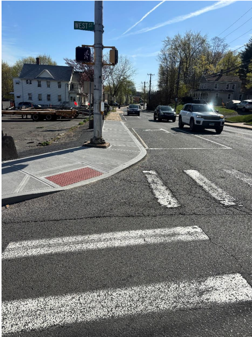
Figure 2: Newly Constructed Ramp - PROWAG Compliant
