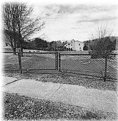
Photo 1: Warner St gate lock missing
