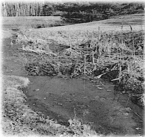
Photo: Sediment and cattails in forebay
