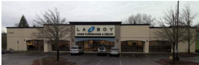
EXISTING BUILDING EXTERIOR
