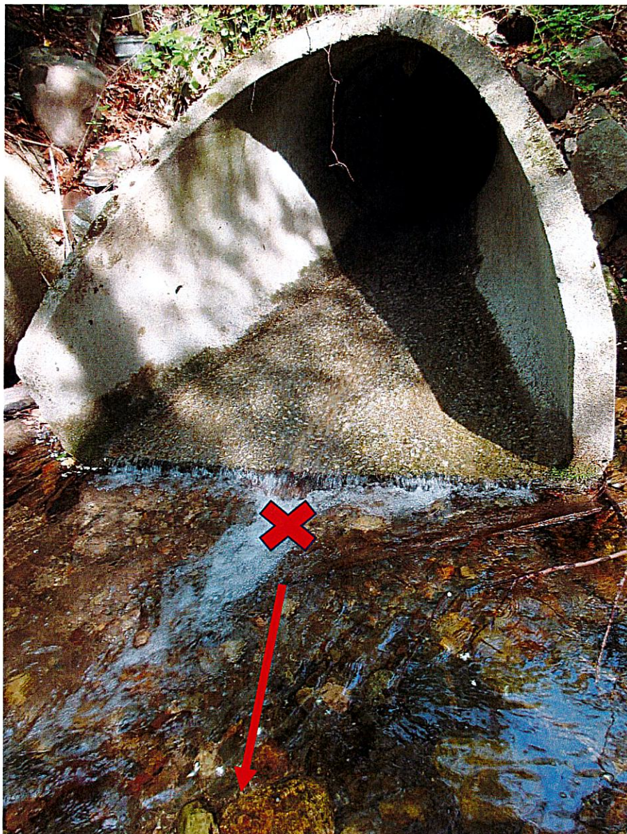
Photo 4a: NPark1 (photo taken 05/28/2025 at approx. 8:55) Unidentified tributary stream flowing through 3 equivalently sized culverts, located on 99 Rockwell Park Rd, Bristol, CT, emptying into the Pequabuck River. Sample point is indicated by a red X. Red arrow shows flow direction.
