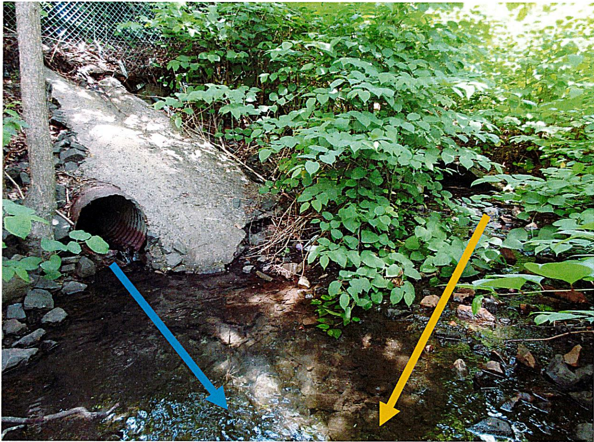
Photo 13b: Greene 1L-1R (photo taken 05/27/2025 during reconnaissance) Photo depicts the confluence between Greene1R stream (blue arrow) and Greene 1L (yellow arrow). Arrows show flow direction.
