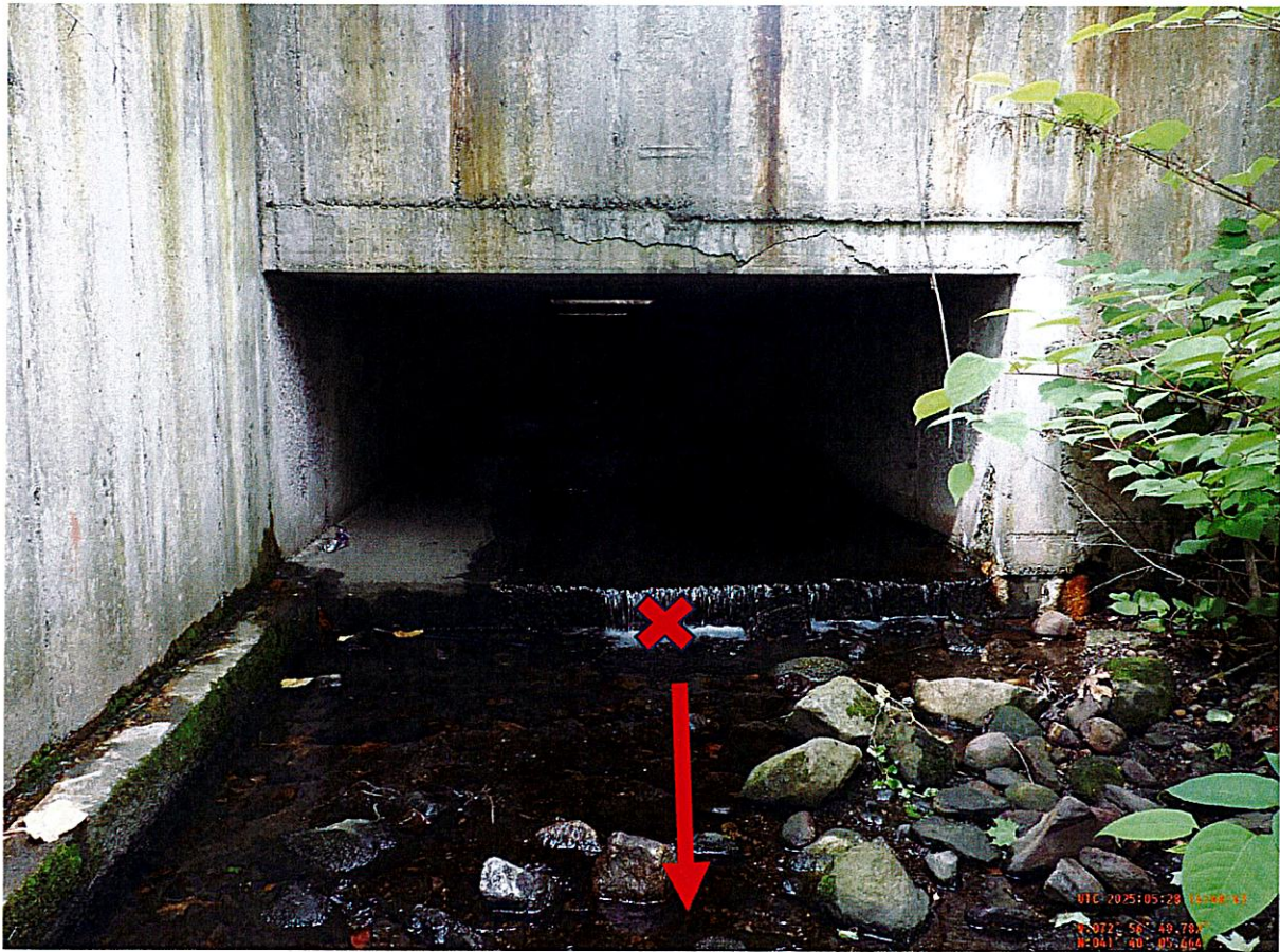
Photo 10a: West1 (photos taken 05/28/2025 at approx. 10:35) Unidentified culverted stream located at 40 West St, Bristol, CT. Sample point is indicated by a red X. Red arrow shows flow direction. Note: Embedded time stamp on photo is inaccurate.
