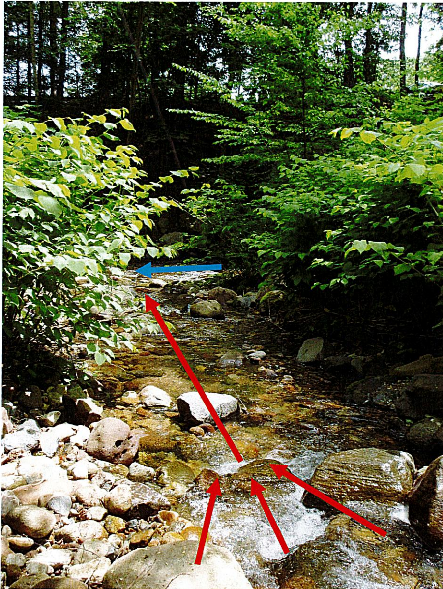
Photo 4c: NPark1 (photo taken 05/27/2025, during reconnaissance) Unidentified tributary stream flowing through 3 equivalently sized culverts, located on 99 Rockwell Park Rd, Bristol, CT, emptying into the Pequabuck River. Photo shown depicts the merging of the tributary stream and the Pequabuck River. Red arrow shows flow direction of the unidentified tributary stream. Blue arrow shows flow direction of the Pequabuck River.
