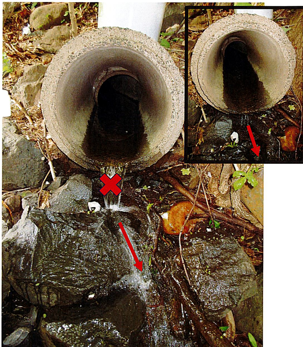
Photo 7a: Gaylord1 (photos taken 05/28/2025 at approx. 9:37) outfall located at 85 Gaylord Street, Bristol, CT, discharging into the Pequabuck River. Sample point is indicated by a red X. Associated photo shows the original flow rate upon arrival, prior to the flow increase and when the sample was collected. Red arrows show flow direction.
