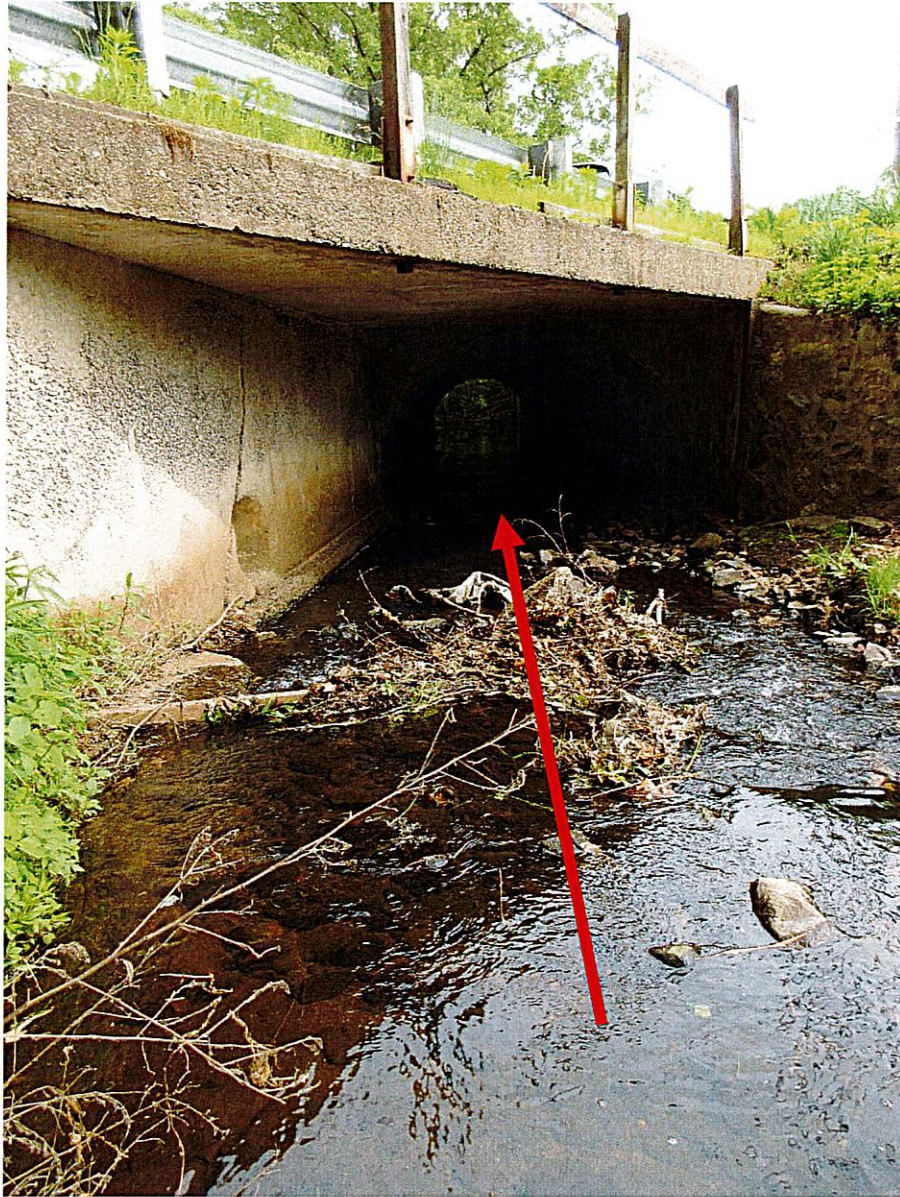
Photo 3b: Mechanic1 (photo taken on 05/27/2025 during reconnaissance) Segment of Copper Mine Brook, running perpendicularly underneath 76 Mechanic St, Bristol, CT, directly upstream of a culvert.
