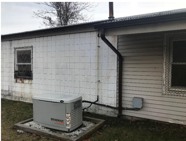
Photo 12-Gas Fired Generator
