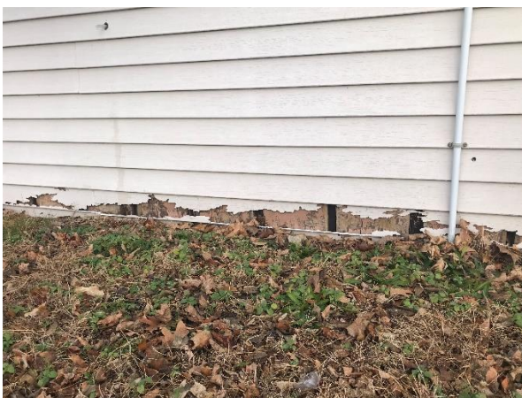
Photo 2-Siding Damage
