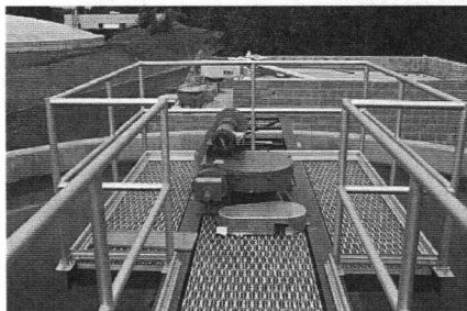
Gravity thickener mechanism and access walkway replacement at Lake Saltonstall Water Treatment Plant
