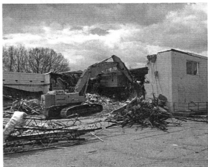
Our in-house asbestos and HBMA group is experienced with abatement and renovation/demolition of renovation efforts when a treatment facility remains occupied and in use.
