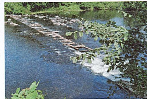
Upon removal, timbers from the dam will be salvaged for research and education.
