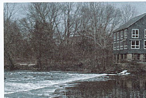
Today, the remains of the dam pose risks to humans and aquatic life.
